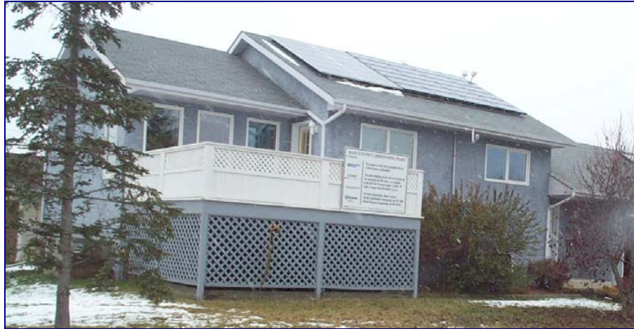
Figure 1. View of Gordon Howell's first solar PV system from 1995 – 2.3 kWdc, 36 solar PV modules, 6 solar PV panels, 3 kWac
